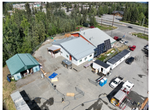
FIDC Fire Station 12 dorm addition, taken 7/7/2026 by Connor Dolan
