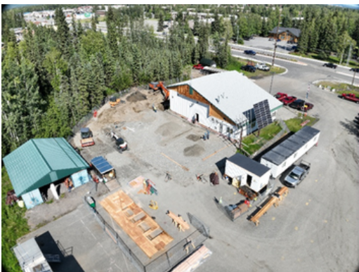
FIDC Fire Station 12 dorm addition, taken 7/31/2025 by Connor Dolan
