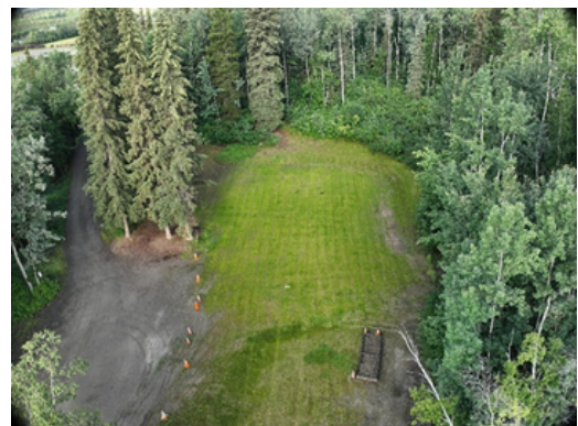
CLHHD Copper Lane Honors House demo, taken 7/21/2026 by Connor Dolan
