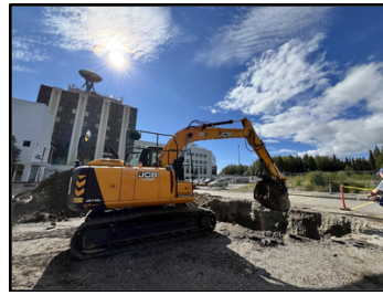
We dug a hold in the WRRB parking lot to address a thermokarst issue and encountered frozen loess at 19' down, a sign that we were getting close to the bottom of the void. photo by N. Platt
