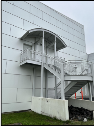
The staircase on the north side of the museum was painted and looks great! photo by N. Platt
