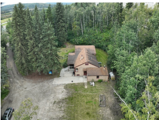
CLHHD Copper Lane Honors House demo, taken 8/18/2025 by Connor Dolan
